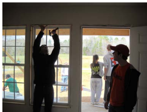
LEFT: Bucknell students install windows in North Carolina home.
