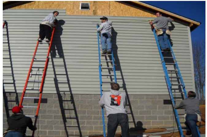
Bucknell students install siding on North Carolina home.
