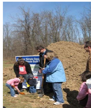
Above: The Lopez family breaks ground.
